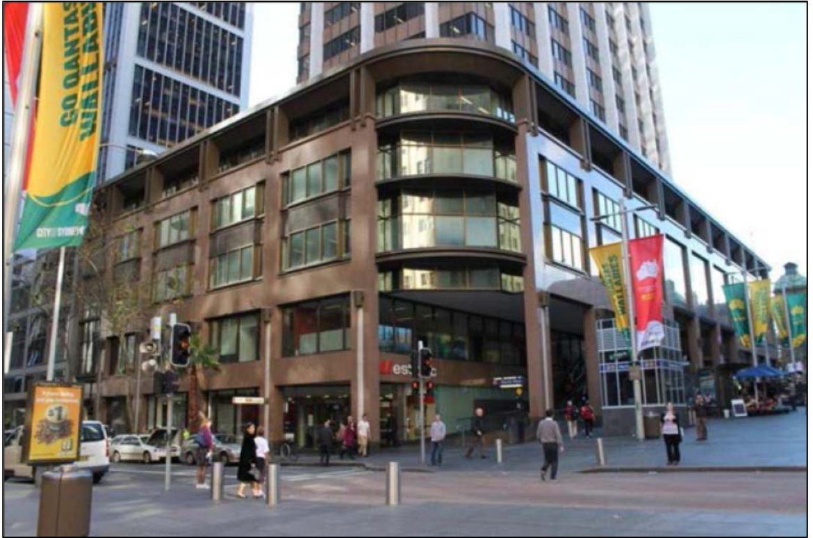
Figure 2 - the podium at 60 Martin Place, looking along Martin Place towards Macquarie Street. Note the poor interface with Martin Place at the ground level, with very low levels of street activity.
